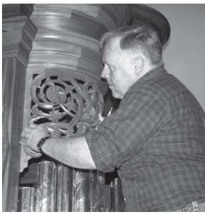
Eric Kenney installs carving
