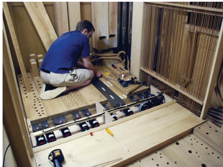
Great organ during installation
