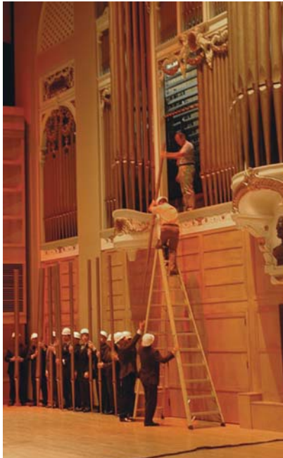
Foley-Baker crew removes façade pipes
