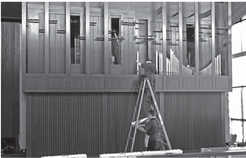
Day 6: After the initial testing of the winding and wiring systems, the pipes are installed. The two ranks visible here are part of the Open Diapason and Harmonic Flute.
