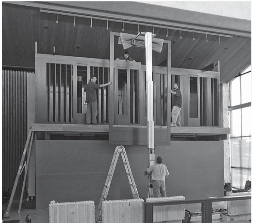
Day 4: With the winding components and blower all in place, the upper casework is hoisted into position.
