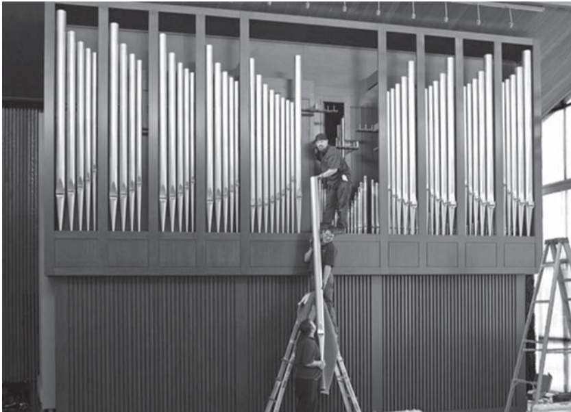
Day 7: The display, utilizing pipes from the Open Diapason, Harmonic Flute and Pedal Principal, brings the organ closer to completion. After tonal finishing, the organ will be used for chapel services as well as diocesan events, all under the leadership of the school's music director, Dr. Thomas Lee.
