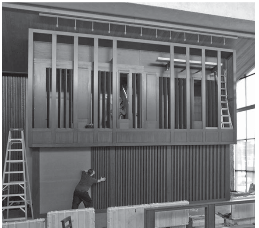
Day 5: The lower case nears completion. Other detail work continues inside the organ, such as connecting chest cables to the relay and winding details.
