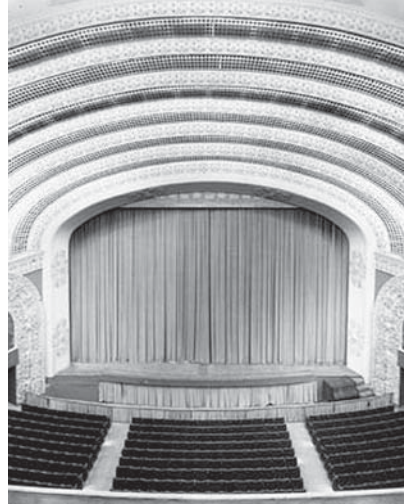
A view of the orchestra section of Temple Baptist Auditorium after the original color scheme was painted over. The organ was installed over the box seating and behind the curved plaster grilles.
