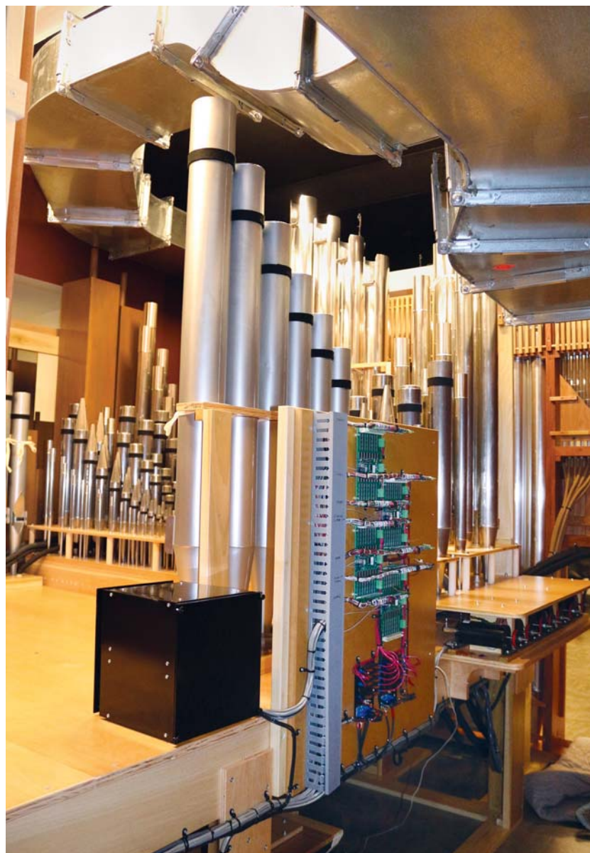
Interior of organ showing low-hanging overhead ducts
