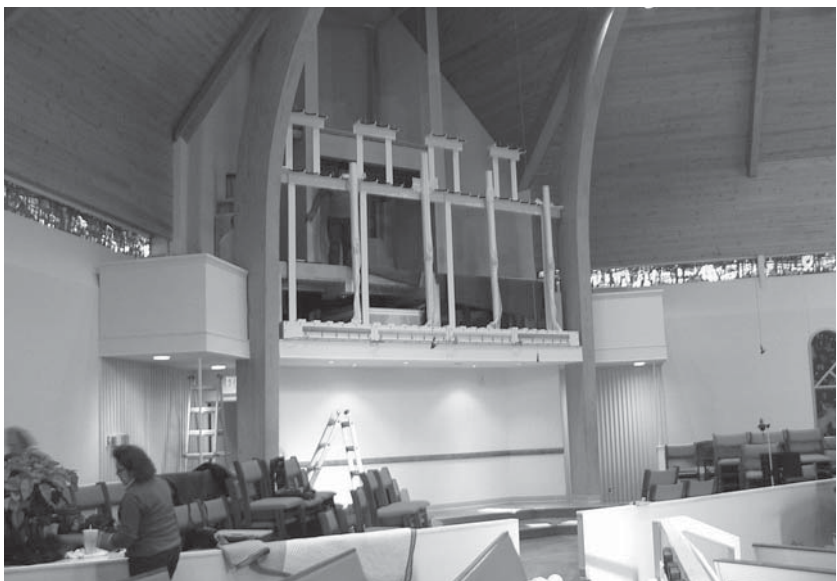
Support racking in place awaiting the 16' Principals
