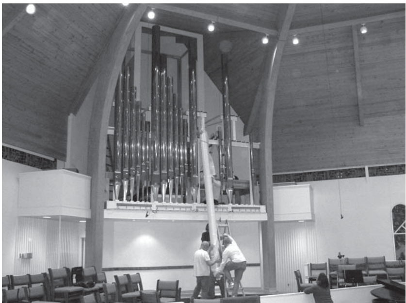
Façade nearing completion
