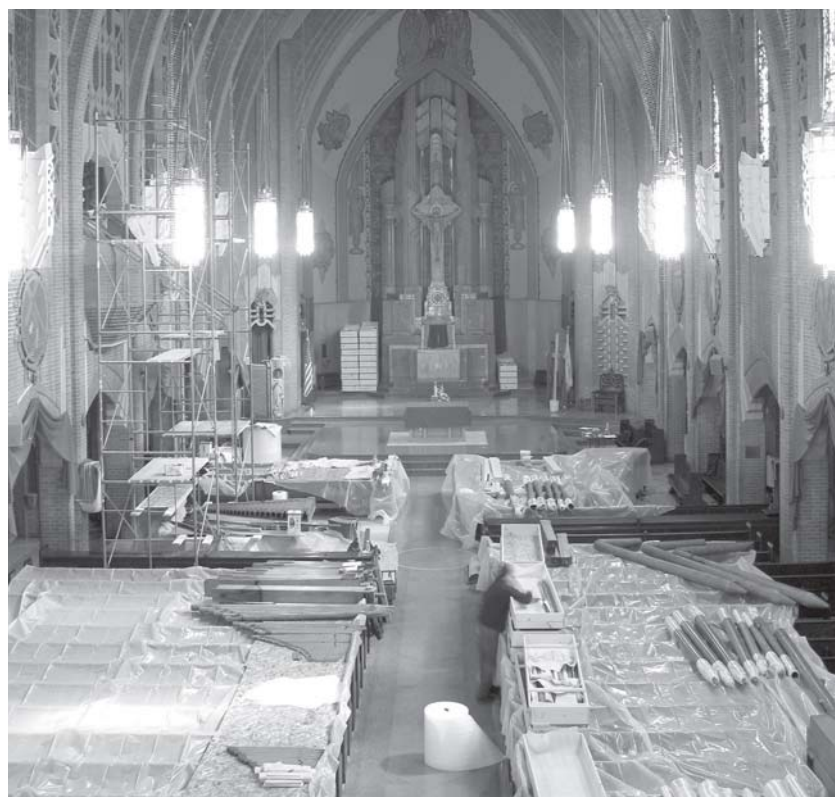
An overview of the church while the Organ Clearing House was removing the organ
