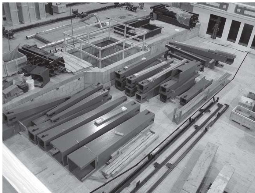
Diaphone staged for installation (photo credit: Louis Patterson)
