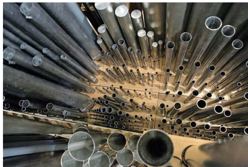
Manual pipes in main case
