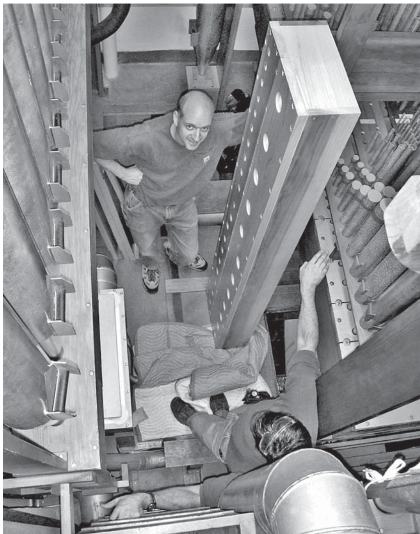
Albert Jensen-Moulton (top) and Joseph DiSalle during installation of the reconfigured Pedal division. Detachable-head reservoir to the left (photo credit: Robert Rast)
