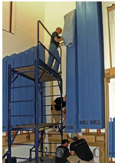
The 32' and 16' basses were mounted on the periphery of the new tower chamber prior to the erection of the main superstructure. The company has painted their large wooden 16' flue stops this Wedgwood blue for years, a practice now adopted by other firms. (photo credit: Sebastian M. Glück)
