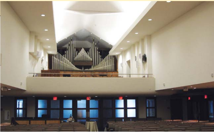
5. An exposed array of pipes in front of a chamber tone grille
