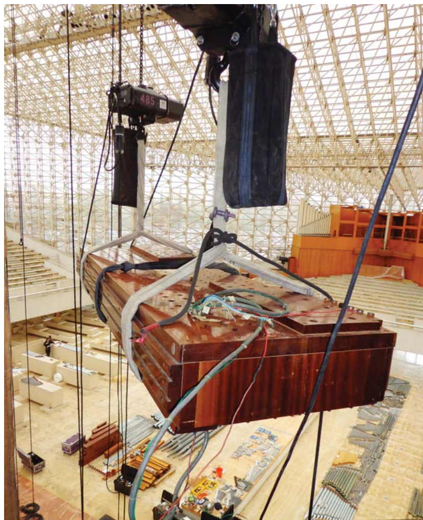
Ruffatti windchests being lowered to floor level
