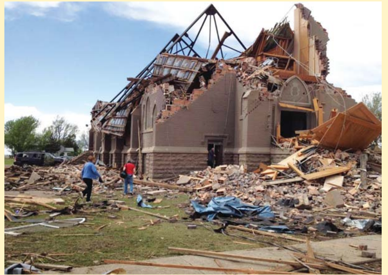
Tornado damage to Zion Lutheran Church
