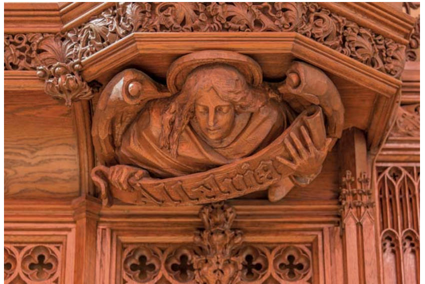
Detail of the 1910 façade woodcarving (photo credit: Len Levasseur)
