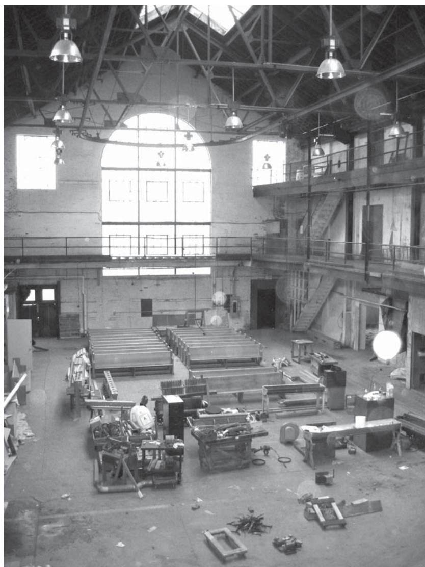
Items brought down from the second floor pipe shop are arranged for placement on one of the ABF trailers, in the world's largest pipe organ erecting room. The large window is visible in the picture of the front of the building. Junchen, vol. 1, has several pictures of the erecting room; in the photo on page 397, the photographer of this picture was standing near the balcony door in the center left of the picture.
