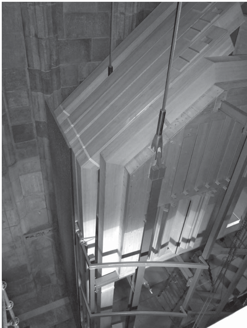
The steel suspension structure
