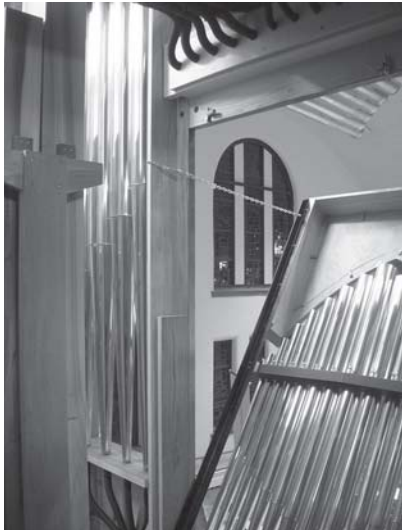
View of en chamade reed access
