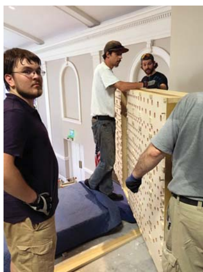
Hoisting main slider windchests
