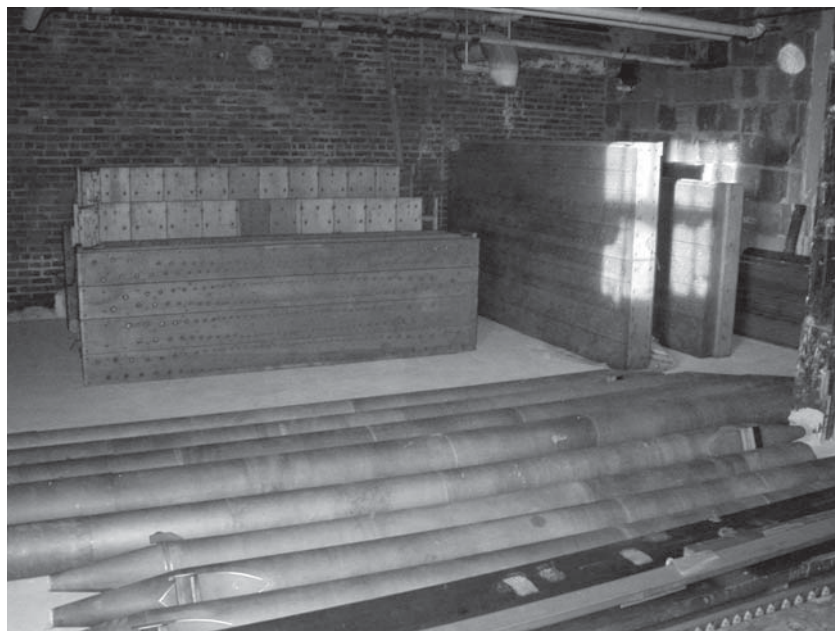
The Left Stage chamber has had all the windchests for the Swell Organ removed to be sent out for restoration. The top photo shows the vertical void created by the chest removal and the lower photo shows the windchests stacked up in a secure room awaiting shipment.
