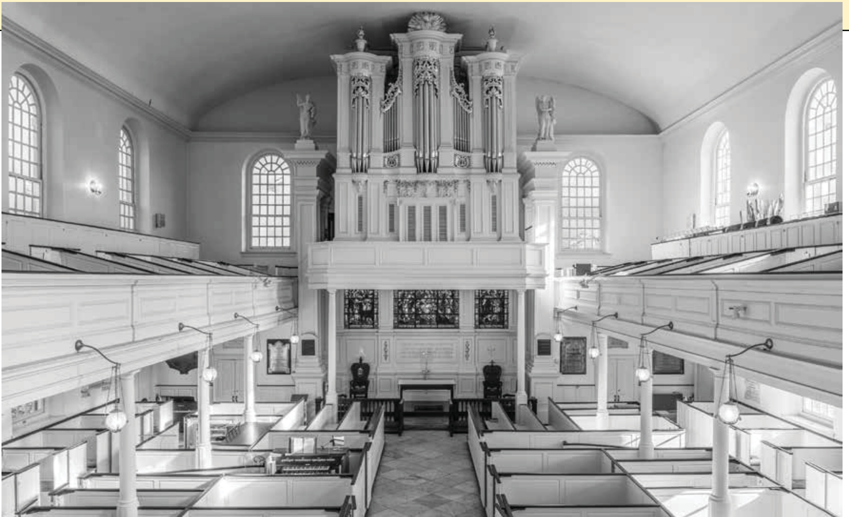
The weight of the Feyring organ proved too much for the original organ loft. In 1797 the large columns and pilasters were added on either side of the loft to help bear the weight, and more strengthening was done in 1805–1806. Sculptor William Rush was engaged in 1807 to carve the two urns atop the side towers. The two life-sized figures (“Exhortation” and “Praise”) and the “Glory” of cherubs peeking over the center tower also were carved by Rush in 1812 for nearby Saint Paul’s Church organ and were presented to Saint Peter’s in 1831 following their removal during remodeling. ©2022 David Ottenstein
