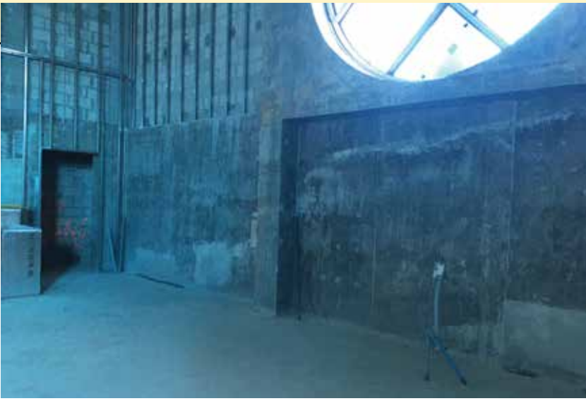
Organ gallery under construction
