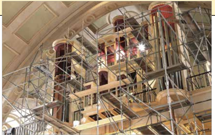
Scaffolding during restoration work
