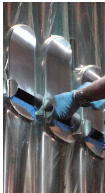
Adjusting façade pipes (photo: Margaret Gettig)
