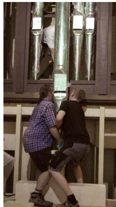
Lifting façade pipes into place (photo: Margaret Gettig)
