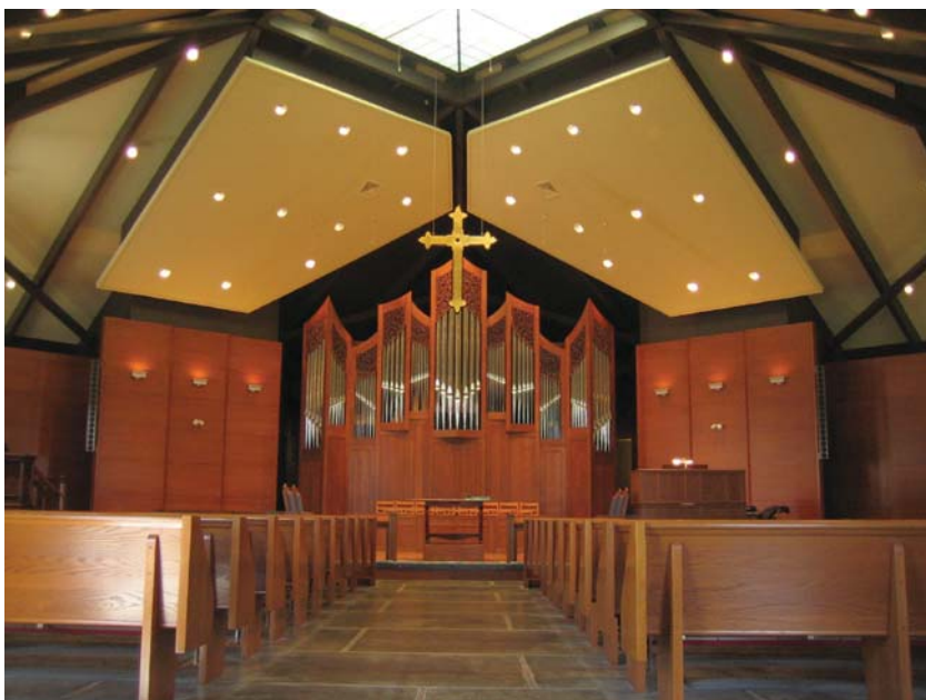
Hard-surfaced floor, wall, and ceiling materials, with sound-diffusing profiles, will help to reinforce sound energy and provide generous reverberation periods.
