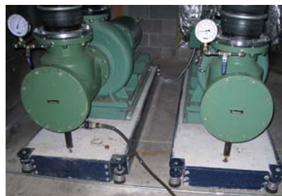
Unwanted noise and vibration can be controlled when equipment is resiliently mounted.
