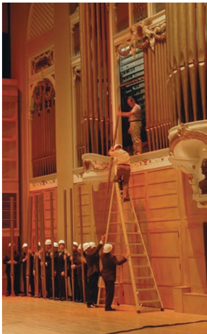
Foley-Baker crew removes façade pipes
