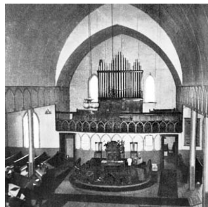
Botwood United Church, Botwood, NL, Forster & Andrews 1928 (photo courtesy Lester Goulding)
