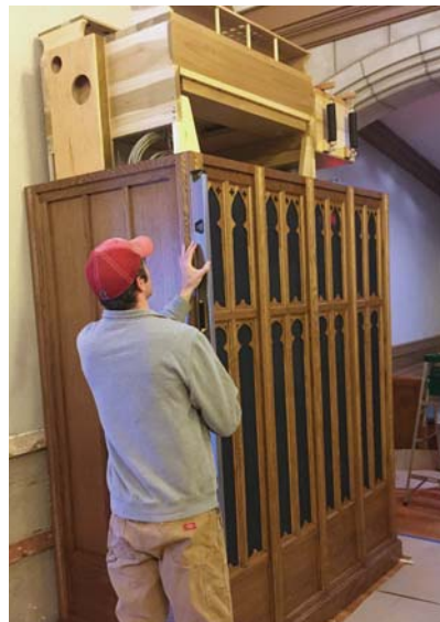
Brian DeWald checks to see if the case-work is level
