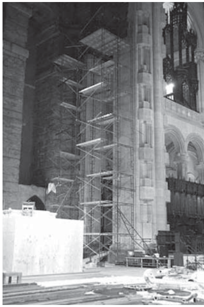
Scaffolding, St. John the Divine
