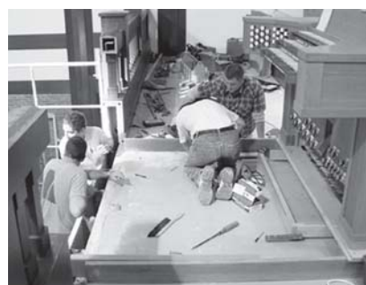
Installation of steel beams to support new Rückpositiv (photo credit: Ron Turner)
