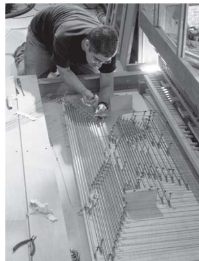
Installation of trackers between Rückpositiv and console (photo credit: Ron Turner)
