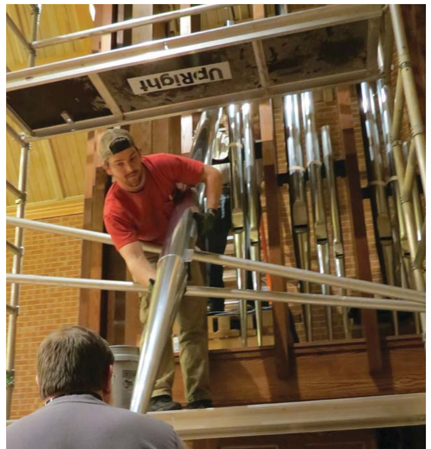
Installing façade pipes
