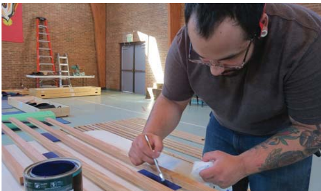
Touching up details of the pipeshades
