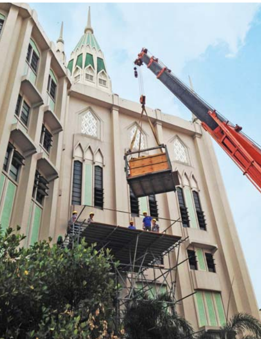
Hoisting console into building (photo credit: Arthur E. Schlueter III)
