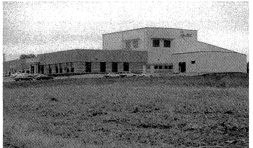
New Reuter corporate headquarters and manufacturing facility
