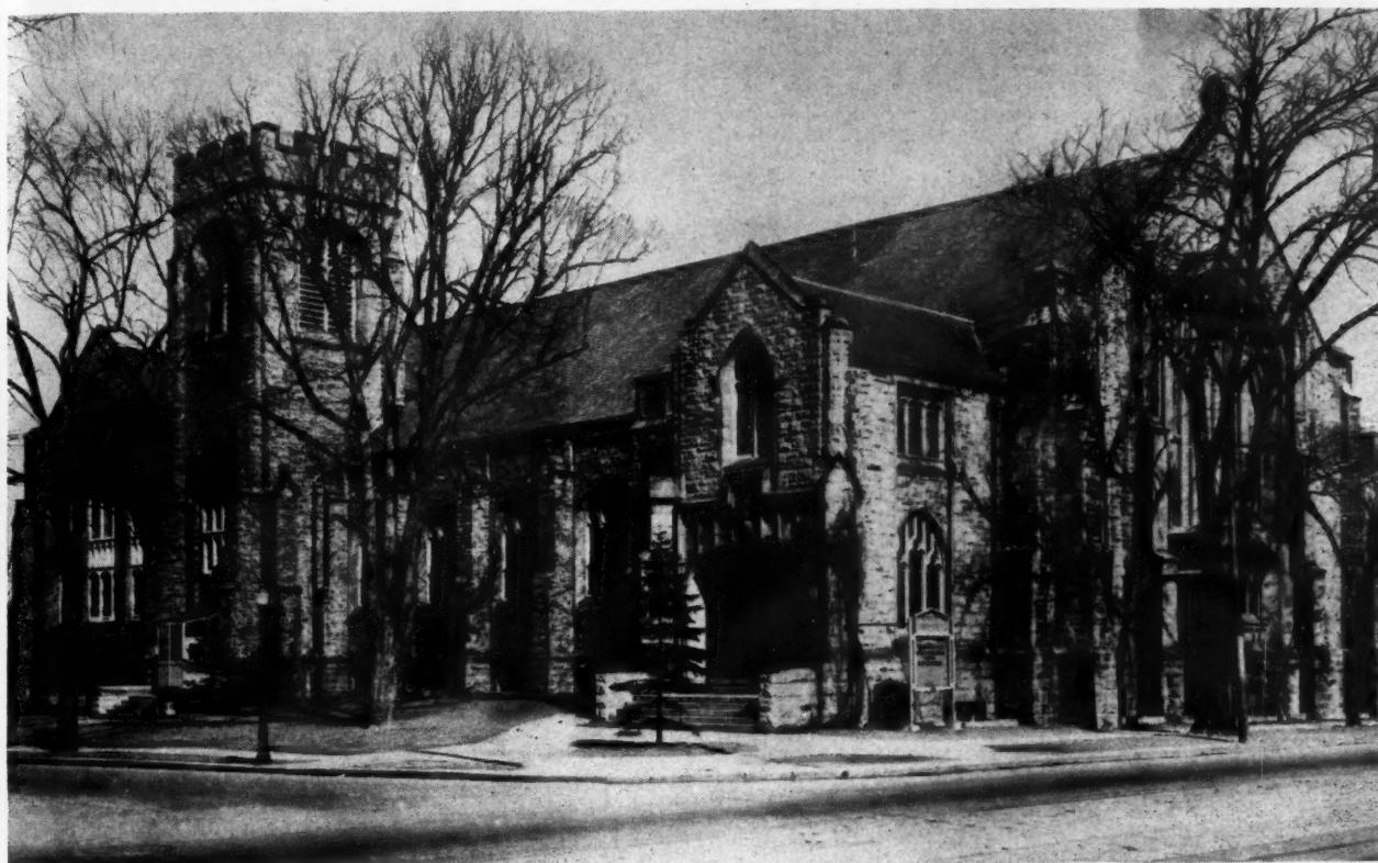
This four manual organ installation will be completed by the Fall of 1956.
